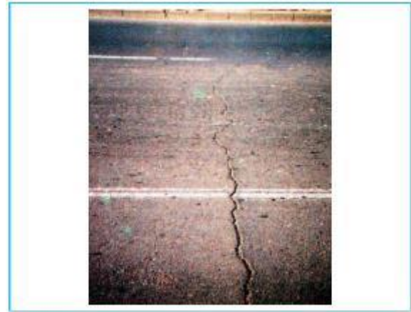
Figure 2 - Fissuration transversale
