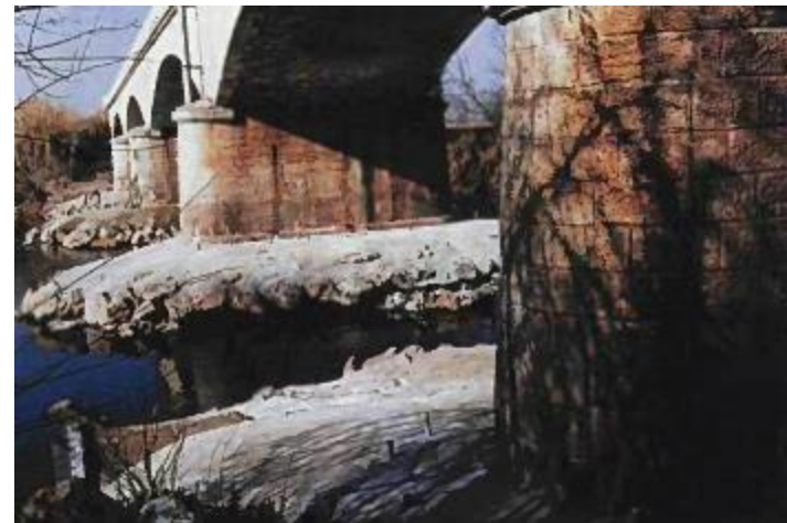
Digging around the piles
