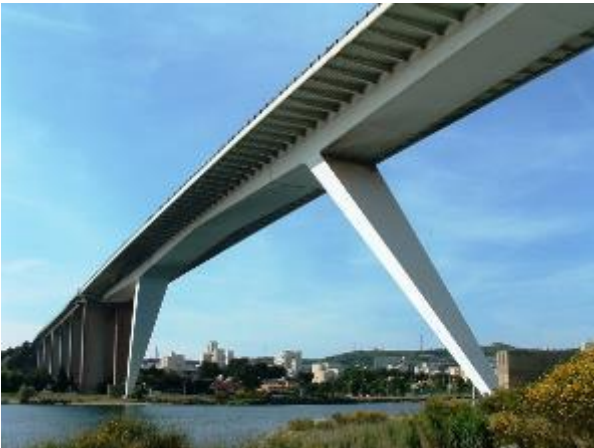
Martigues Viaduct (France, 1972) Length 300m, main span 130m.
