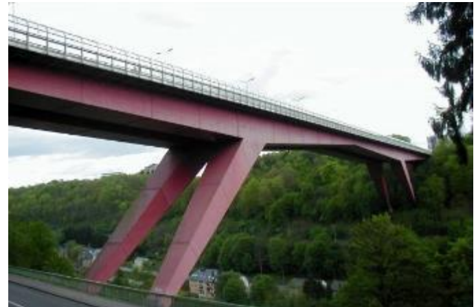
Grand Duchess Charlotte Bridge (Luxembourg, 1965) Length 355m, height 74m, main span 234m.
