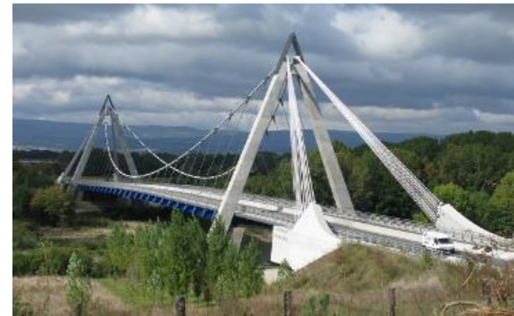
Grand bridge on the Loire (France, 2008)
