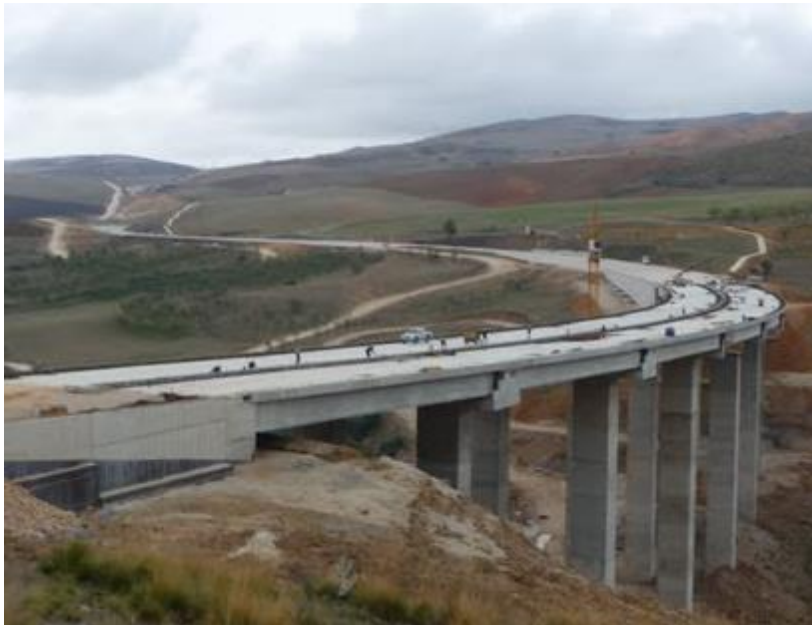
Bridge on the East-West highway ( Bouira )
